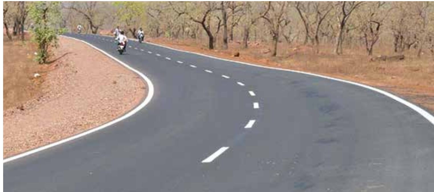
Khadim-i-Punjab Rural Road Programme, a flagship project of Muhammad Shehbaz Sharif under which farm-to-market roads spanning over thousands of kilometers were constructed across the province
